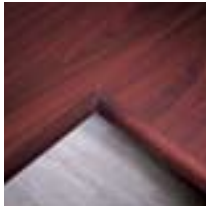
Reverse Coped Edges & Common Grain Direction
